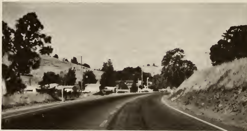
Figure 53 Driver View - 1200 Feet (366m) (Amador Central Crossing)
